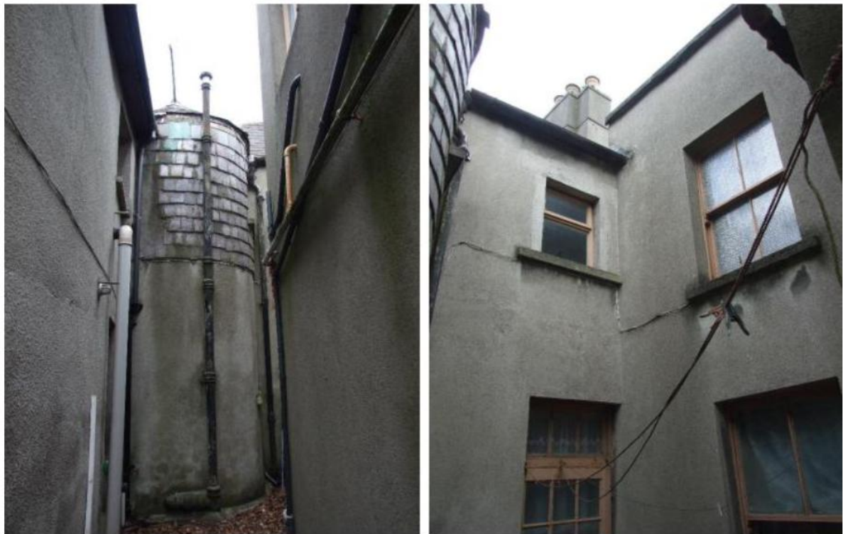
Turret addition / Internal yard to north
