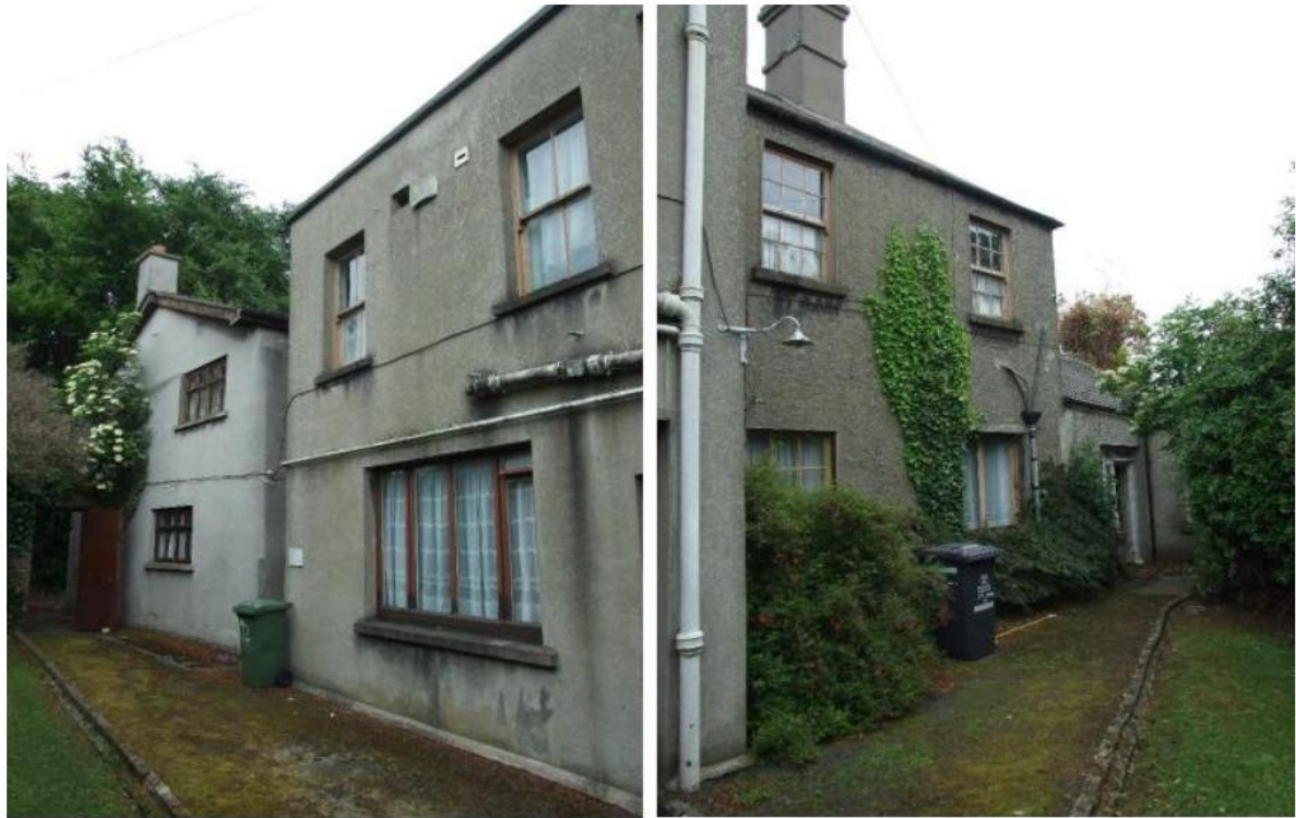
Rear (north) elevations
